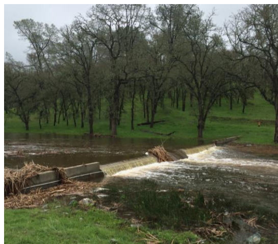
Water is moving well this year through a flow-measurement weir on Littlejohns Creek. Computer-managed valves control Skyrocket Lake water discharge.
